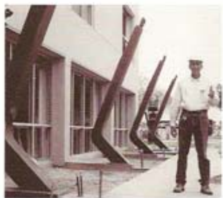
Salvaged dozer stabilizer arms provide support for a garden awning structure. Site lighting bollards were designed for the Empire project and utilize fluorescent lamps in amber globes. Bill Tonnesen is pictured lower right.
