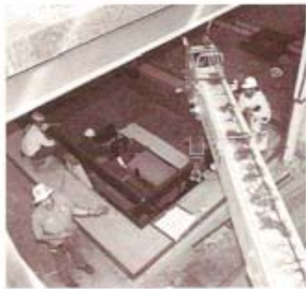
An antique bulldozer, on display in the original lobby, was installed under a glass floor in the new boardroom. It is surrounded on all sides by backlit glass walls. The floor joists are also glass.
