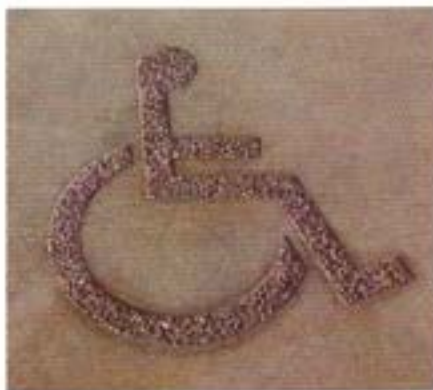
Twin pools with stainless steel D-10 dozers spill water beneath an entry bridge. Copper ore was used for landscaping and parking symbols are sandblasted rather than painted.
