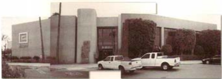
The original elevation was largely blocked by overgrown shrubbery, a stair tower, dark glass, and parked cars.
